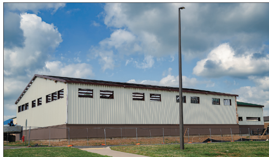
New gymnasium under construction.
