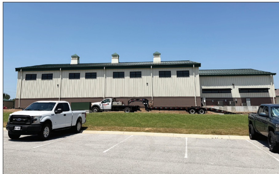
New Fitness Center Gym nearing completion.
